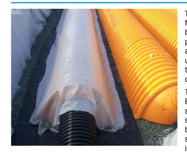
An important component of any Stormwater Pollution Prevention Plan is inspection and maintenance. The StormTech Isolator Row is a patented technique to inexpensively improve stormwater quality and provide easy access for inspection and maintenance. By using the StormTech Isolator Row a TSS removal of 80%, a hydrocarbon (diesel) removal of 90%, a total Zinc removal of 53% and a total Phosphorus removal of 49% can be achieved.\*
