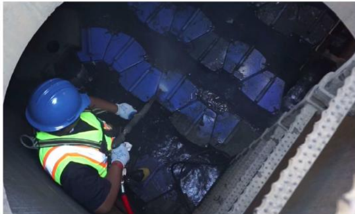
Power washing of Up-Flo Filter components
