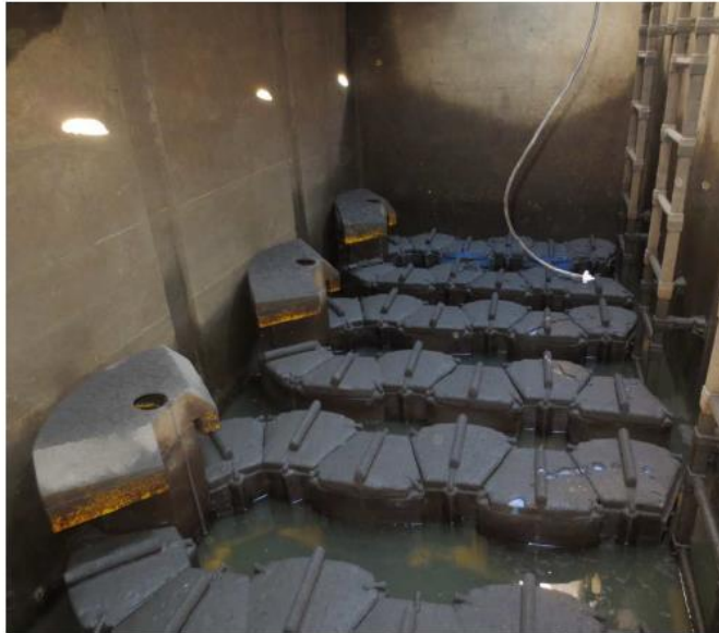
Power washing of Up-Flo Filter components
