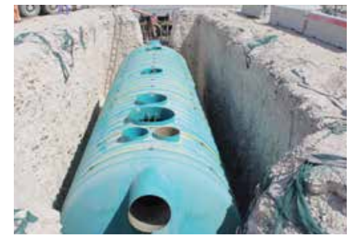
Al Rayyan Road Support - Qatar
