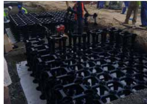
Butterfly Building – Dubai Internet City
