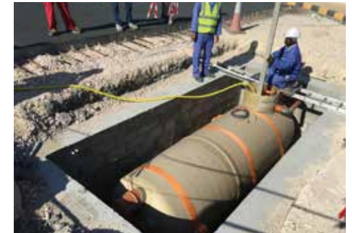
Woqod Station - Qatar
